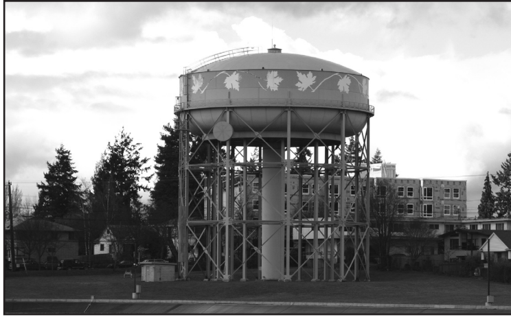
• The Maple Leaf water tower & reservoir near Roosevelt and NE 85th •
